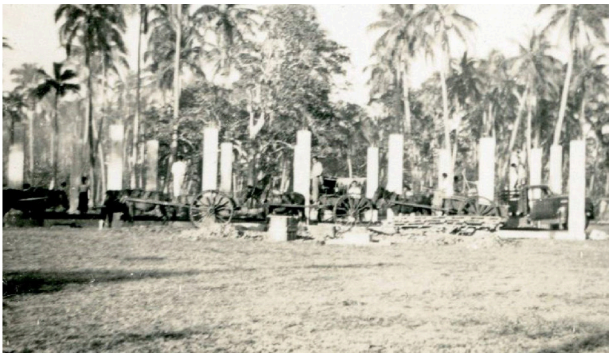
St. Joseph's Chapel as it was being built with chariots and horses until opened in April 1953. College truck on the right was shipped from NZ in parts for Fr. Wall to assemble at 'Api Fo'ou
