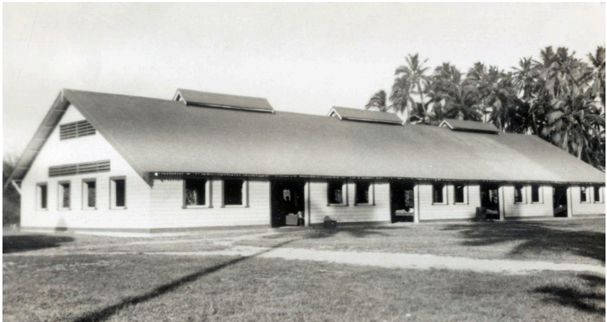
St. Joseph's dormitory, completed in 1949 and later used as classrooms, was built by Lemoto Ongolea, aided by skilled students from Vava'u and the Niuafo'ou evacuees living at Matāliku
